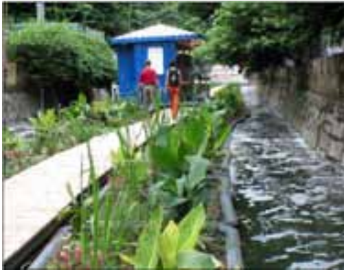
Figure 13: Image of Restorer in Baima Canal, China. Restorers can either be free-floating or linear.
