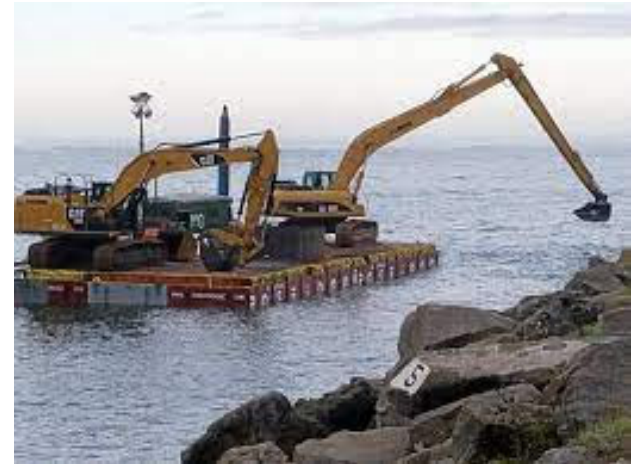
Dredging & Dredge Spoils
