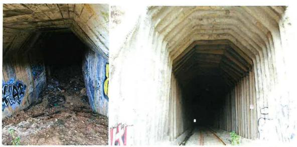
Ph 3033 Tunnel 6 - Burned/Collapsed
