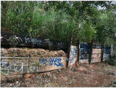
Ph 3037 Failing wall at Tunnel 5
