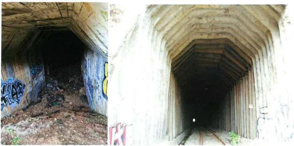
Ph 3033 Tunnel 6 - Burned/Collapsed
