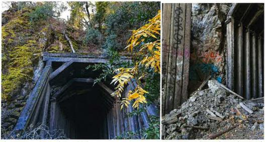
Ph 2806 Tunnel 9 North Portal failure
