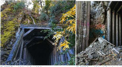
Ph 2806 Tunnel 9 North Portal failure
