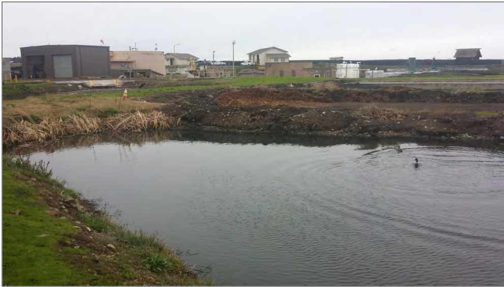
Figure 13. Western Sludge Pond. The western sludge pond had more wetland vegetation in and around the pond edges, although it is annually cleared.
