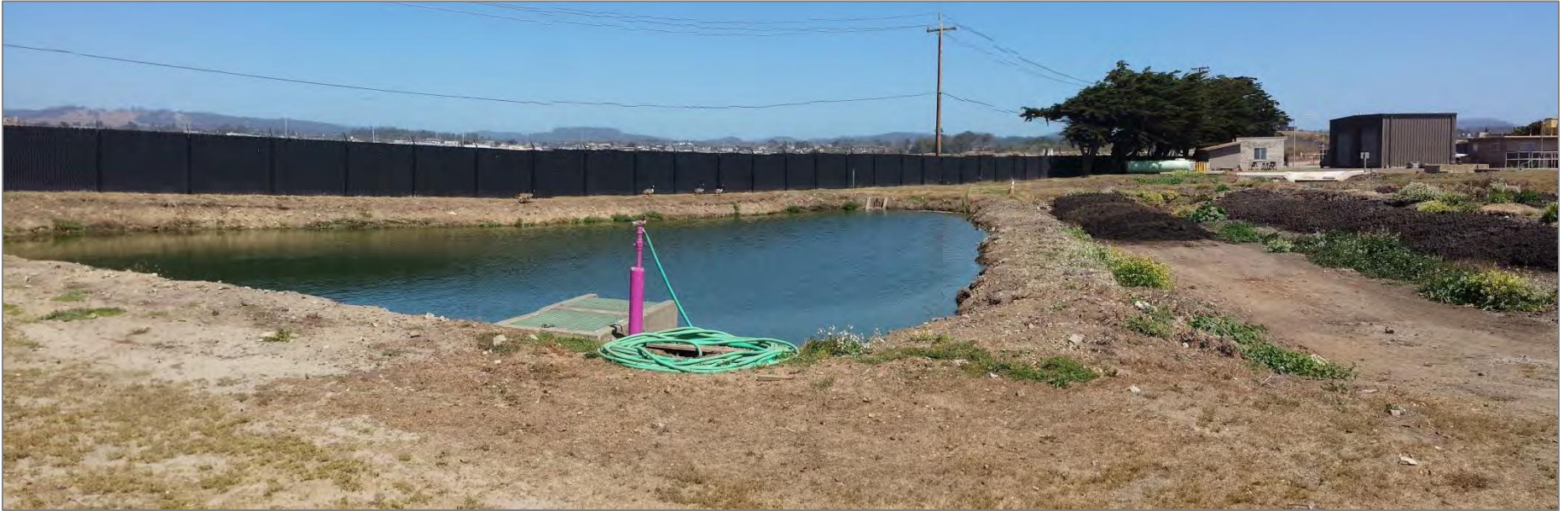
Figure A-2. Northeastern View of the Western Sludge Lagoon.
