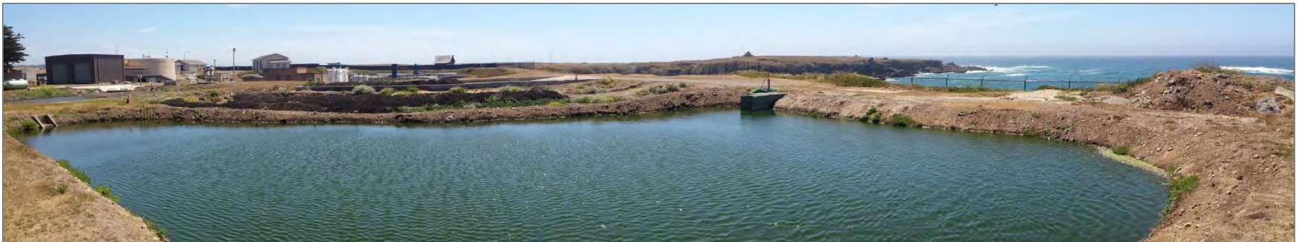
Figure A-3. Southwestern Panorama of the Western Sludge Lagoon.
