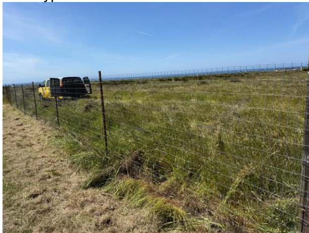
Photo 3: Site fencing near Cypress Street entrance and Coastal Trail (photo direction: west)
